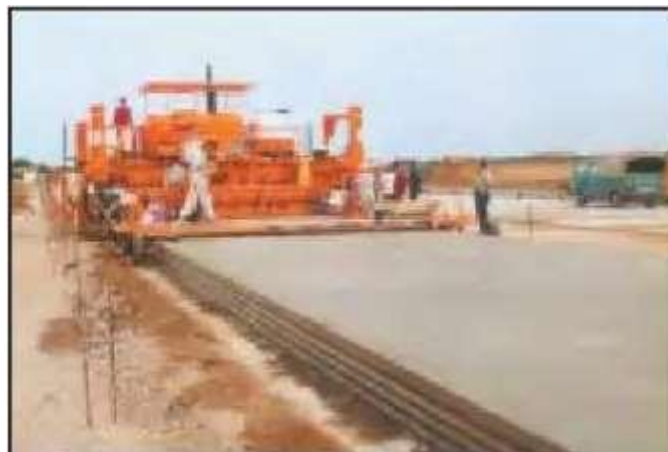
Fig-6 placing of concrete
