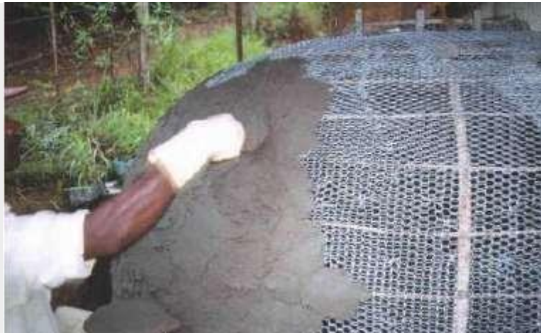
Fig-14 ferro concrete
